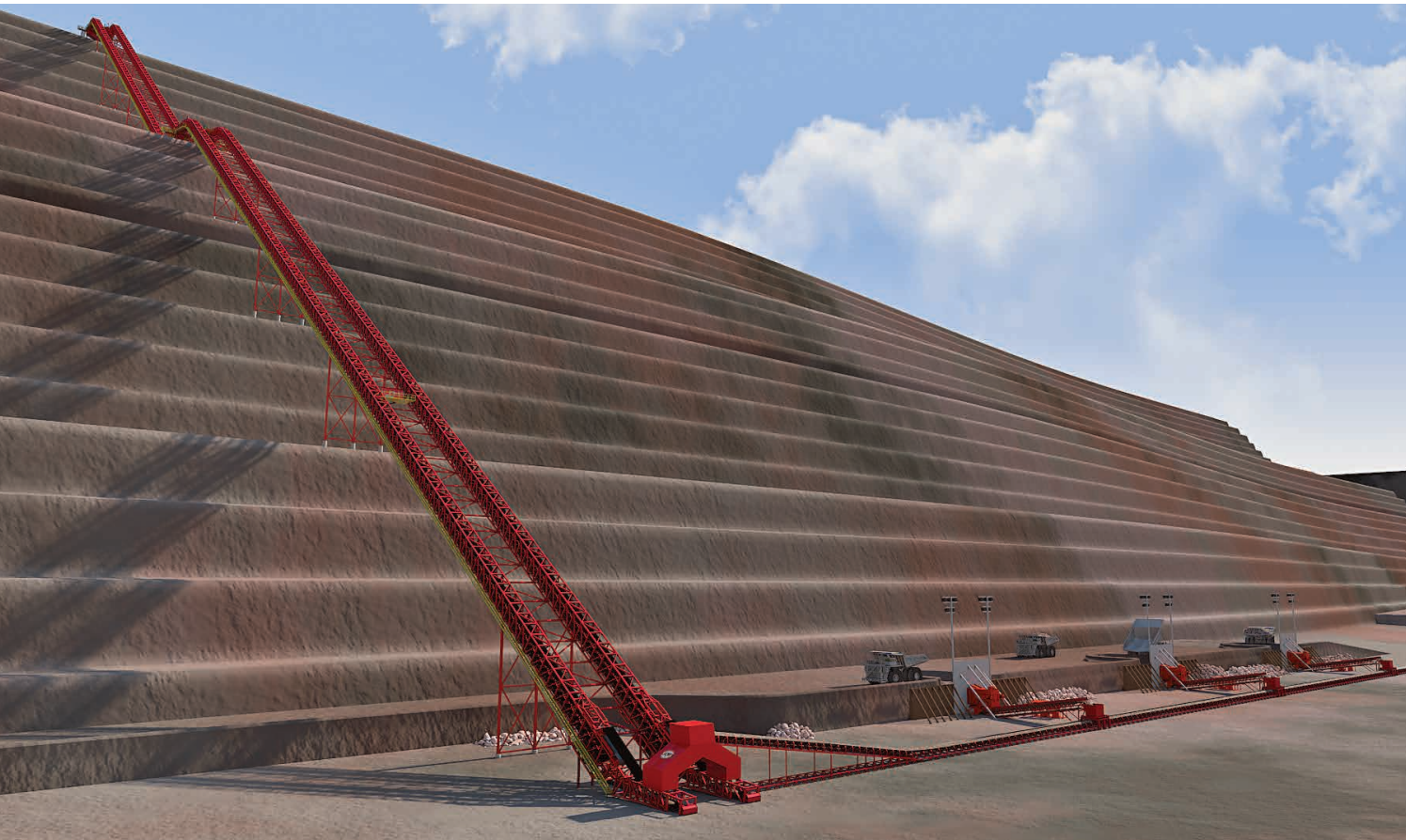
Joy feeder breakers and sizers are utilized to process material in the pit. HAC systems elevate material from the pit onto overland conveyors for processing.
